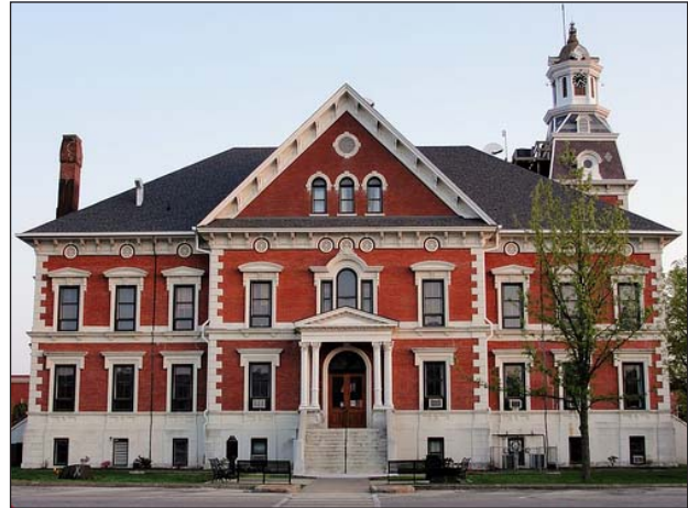
McDonough County Courthouse, Macomb, Illinois (present day)
